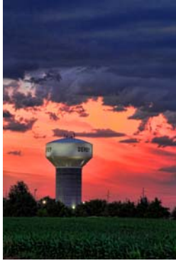
The north Rock Road water tower after a storm.
