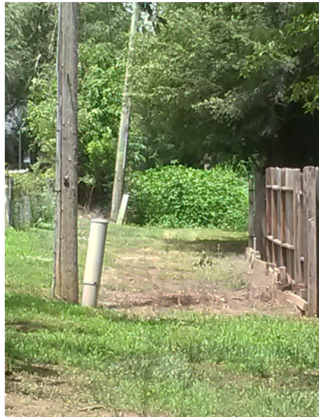
This shows an example of a well-maintained portion of an easement and an area that is not well-maintained.
